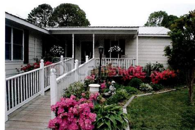
Photo of home with lovely wheelchair ramp
