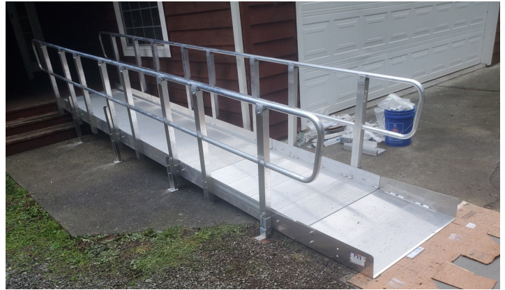
We installed this ramp!
